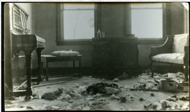
War damage at Shanghai Sanitarium, 1949
